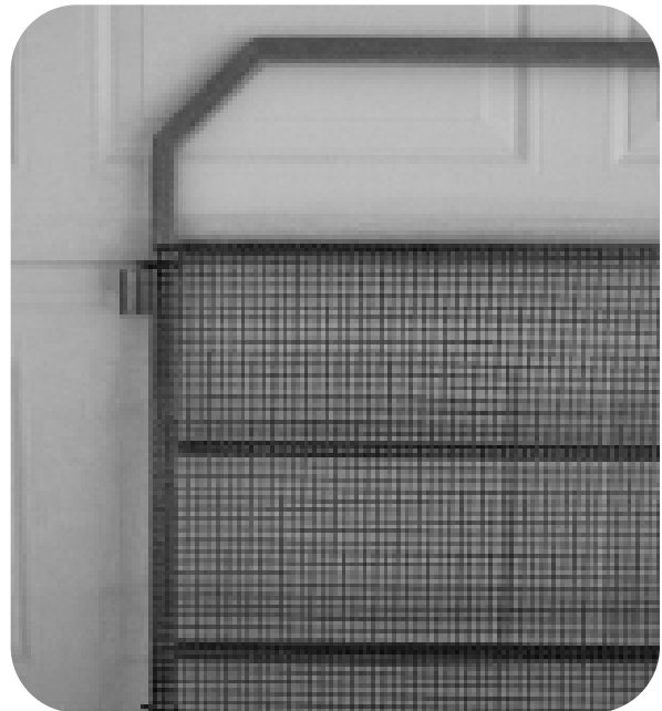
Mesh Fencing attached with zip ties.
