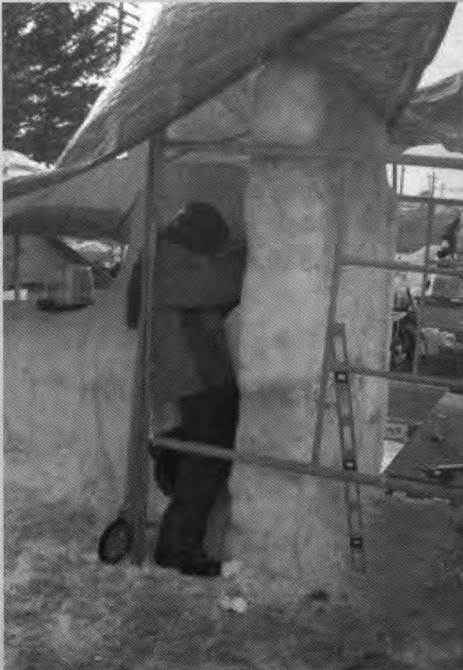
Russ working under the tarp on a very windy day three.
