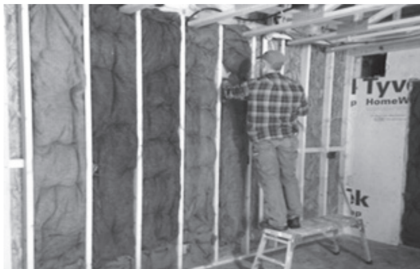
Alpaca insulation was easily installed in one of the barn-like structures on Alpaca Spring Valley Farm in Minerva. The product is easy to cut, soft and not all prickly. Alpaca Spring Valley Farm
